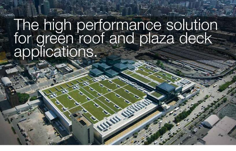
New York's Jacob K. Javits Convention Center features a 5,000-square green roof assembly that includes Siplast NVS Lightweight Insulating Concrete, Paradiene 20 HV TG, Teranap, pavers, and Paraguard Coping.
