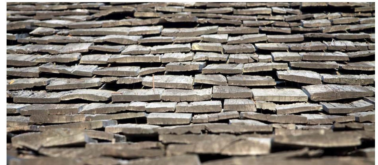
Pictured: Shake products showing warping, curling and mold growth
