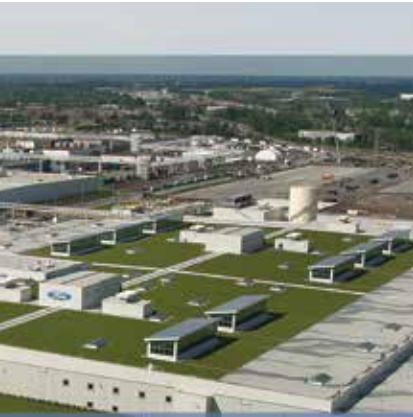
▲ Siplast Teranap was installed on this automobile manufacturing facility in Michigan, creating the largest green roof in North America.
